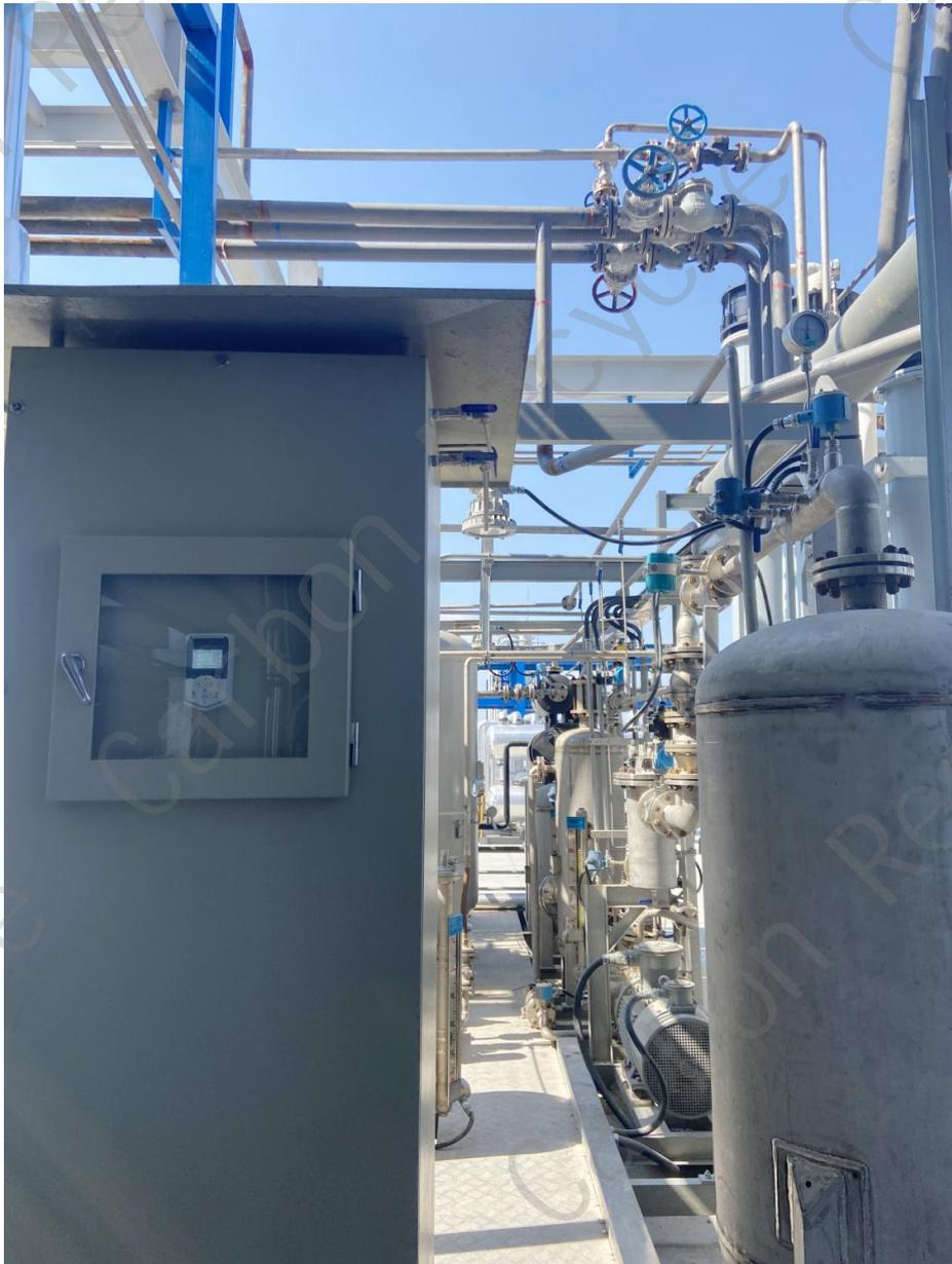
**Fig. 19:Photo of 100Nm<sup>3</sup>/h Petroleum ether solvent recovery equipment on site**
