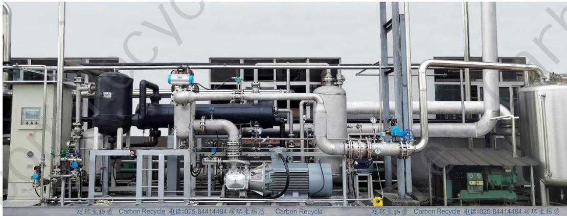
**Photo of 800Nm<sup>3</sup>/h Dichloromethane gas recovery equipment on site**
