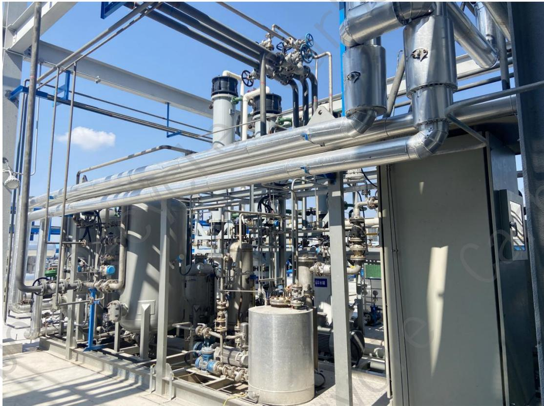
**Fig. 7:Photo of 600Nm<sup>3</sup>/h propylene oxide solvent recovery equipment on site**
