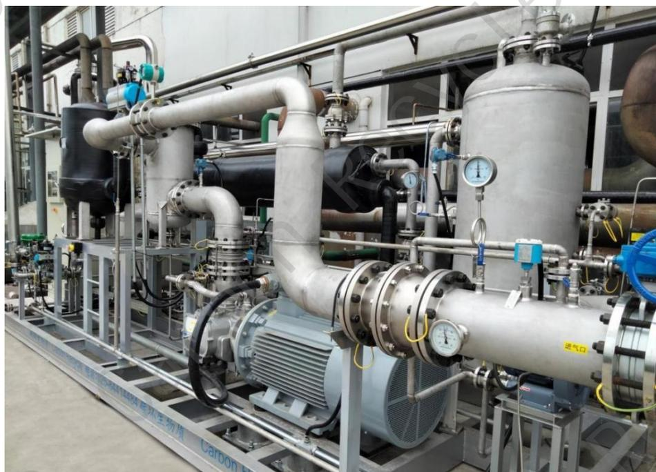
Fig. 1:Photo of 500Nm<sup>3</sup>/h Propanone waste gas recovery equipment on site
