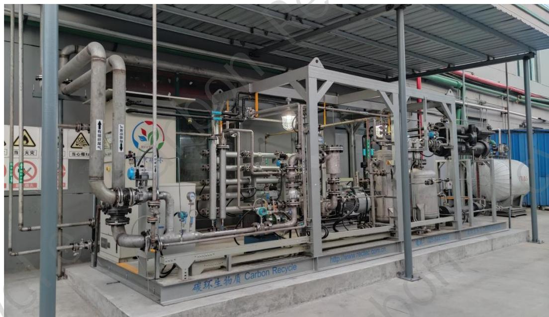
**Fig. 8:Photo of 300Nm<sup>3</sup>/h methyl tert-butyl ether (MTBE) recovery equipment on site**
